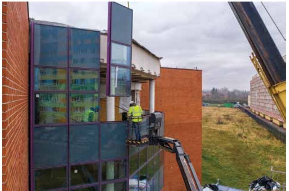
Figure 1: EENSULATE module installation at the Polish demonstration site
