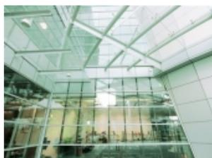
Curtain wall facades are structures that span multiple storeys, and are normally made of metal elements and glass surfaces that bear only their own weight and no other dead load weight from the building.
